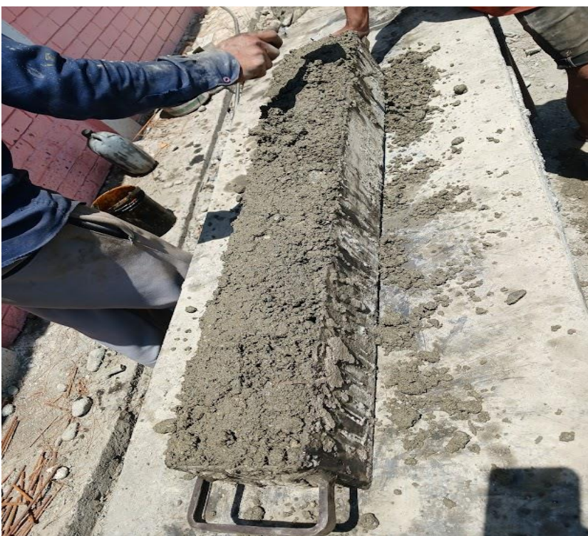
Preparation of boundary pillars for Boundary Demarcation
